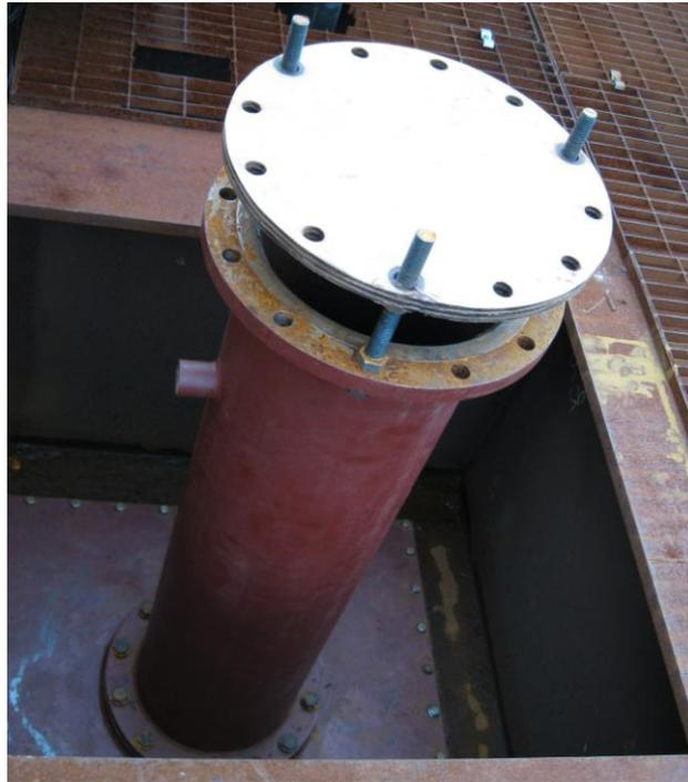
Figure 4: A 300 mm diameter chimney fitted to the top of the tank, showing the hydrogen sensor connection boss and the wooden cap.
